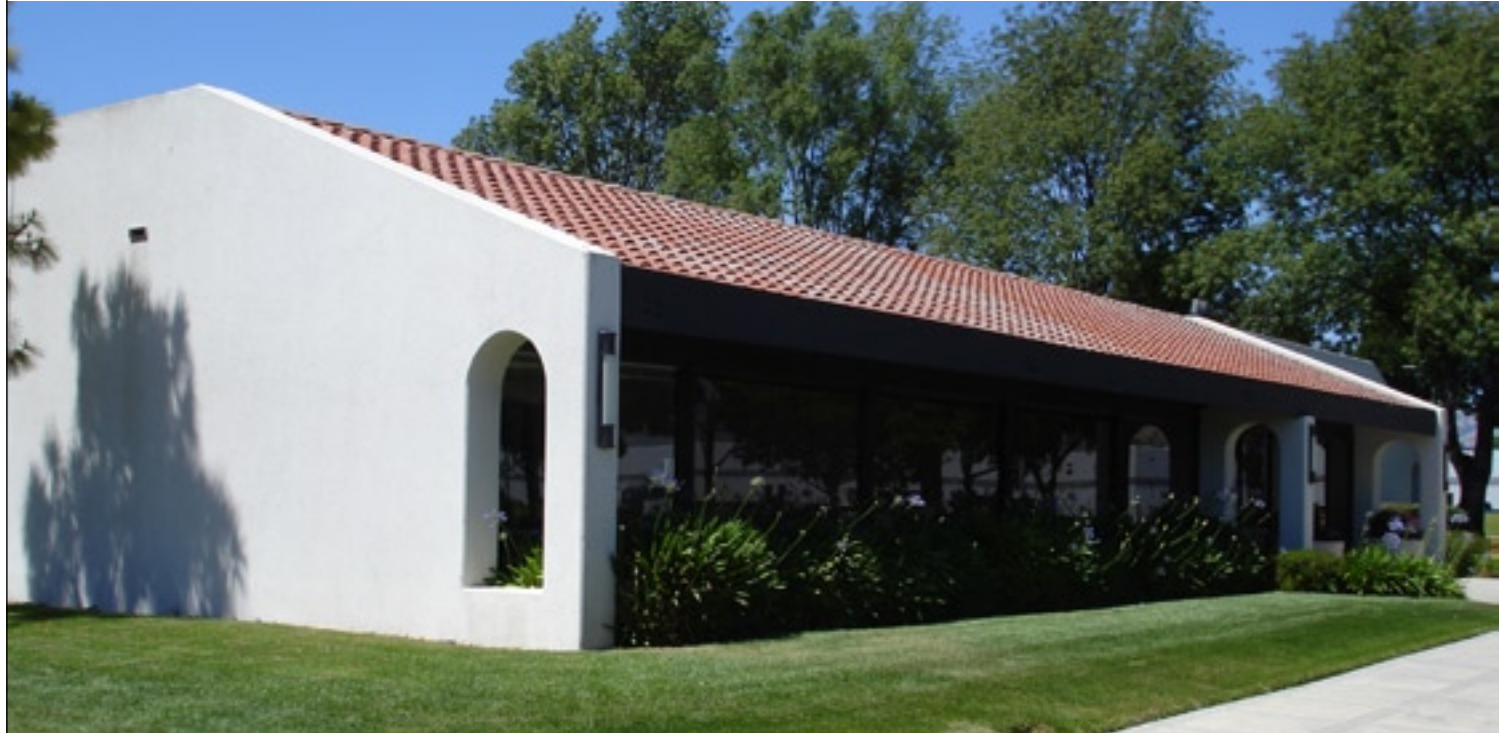
2121-2125 ZANKER ROAD SAN JOSE
